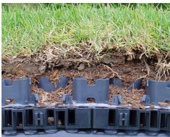
Consider using grass paver type product to stabilize the path to Mt. Hoy
