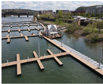
New floating dock with finger piers
