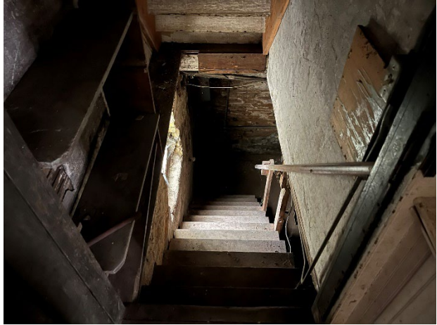
Figure 71. Wood stair leading to basement.
