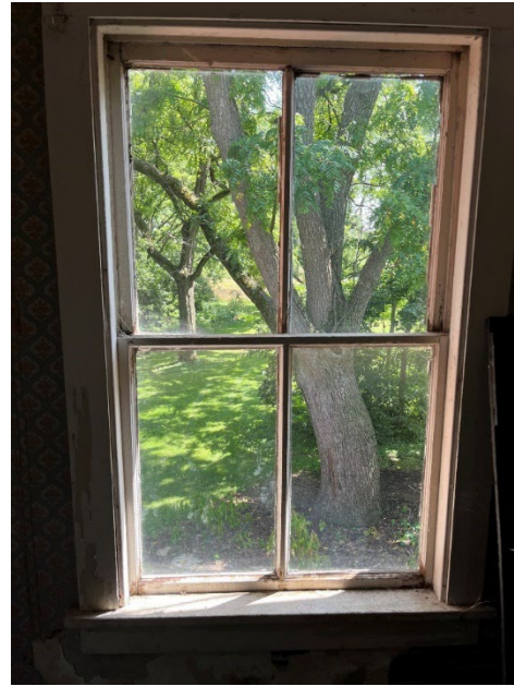
Figure 63. Two-over-two double-hung windows at second floor.
