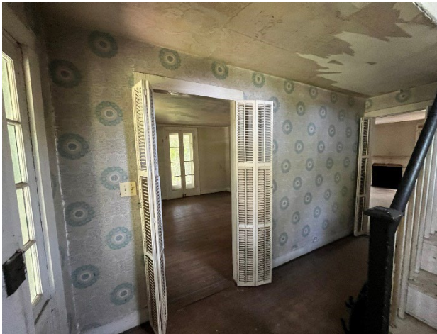
Figure 29. Louvered wood bifold door leading to parlor.
