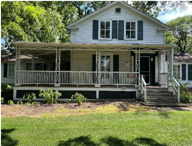
Figure 19. North facade of Oak Cottage.
