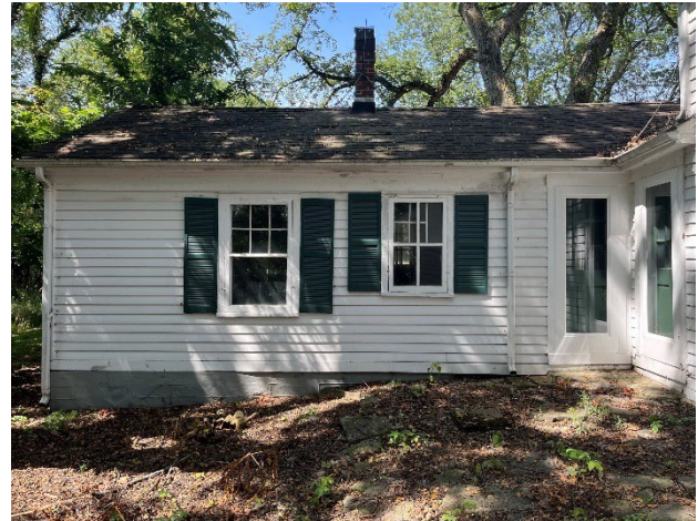
Figure 26. East facade of the west wing.
