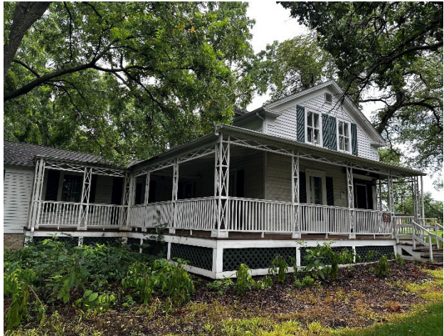
Figure 10. Wrap-around porch at north elevation.
