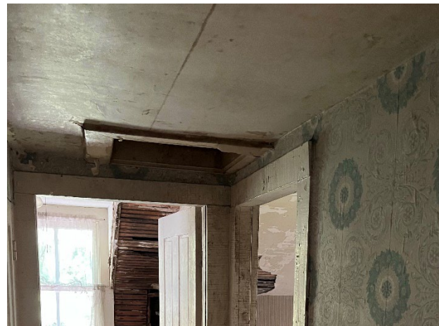
Figure 65. Wood access hatch in hall leading to attic.
