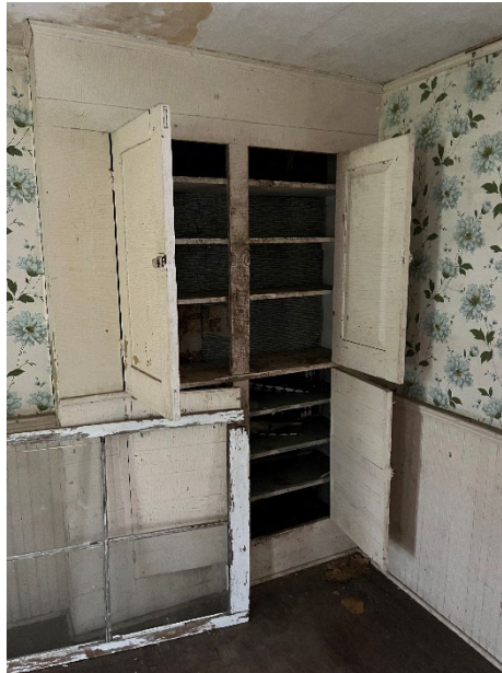
Figure 47. Built-in wood cabinets at east wall of dining room.
