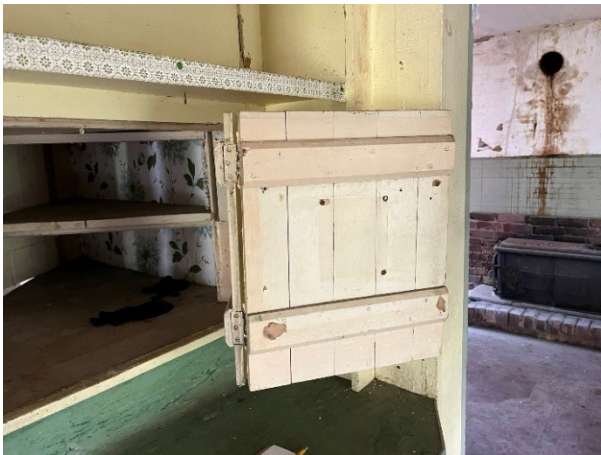
Figure 56. Through passage cabinet from kitchen to dining room.
