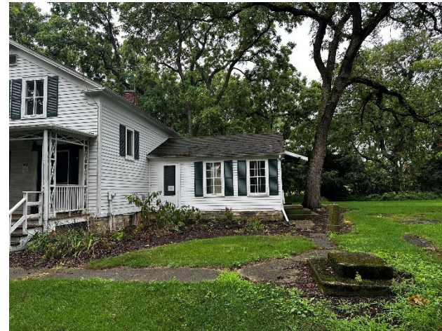
Figure 5. Concrete-paved walks and concrete mounting block (at right) adjacent to house.
