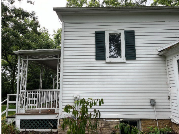
Figure 22. North end of the east facade of the main house.
