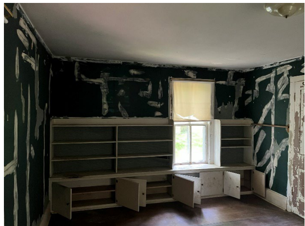
Figure 45. The east room with built-in cabinets along the south wall.
