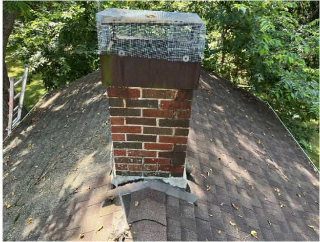
Figure 14. Brick chimney at west wing.
