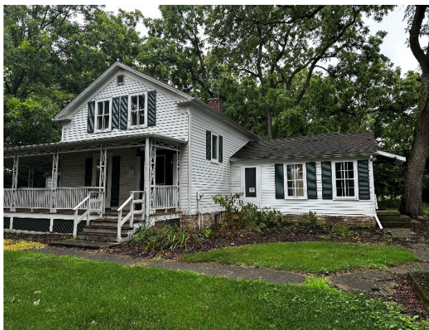
Figure 7. Partial north elevation of Oak Cottage.
