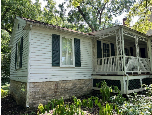
Figure 23. North facade of the east wing.
