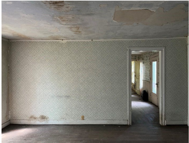
Figure 40. Wood door leading from living room to west wing.
