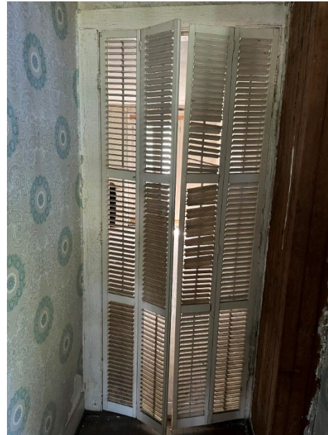
Figure 30. Louvered wood bifold door leading to living room.
