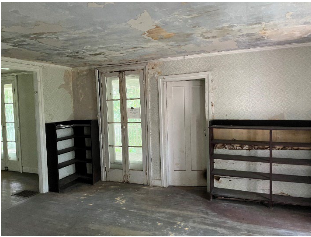
Figure 41. Wood door leading from living room to east wing.
