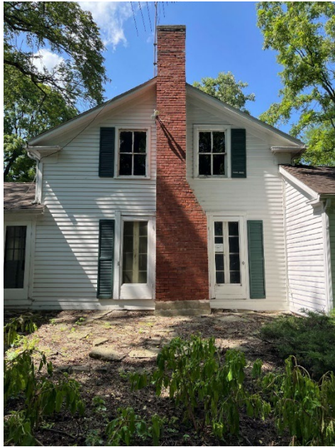
Figure 13. Brick chimney at south elevation.
