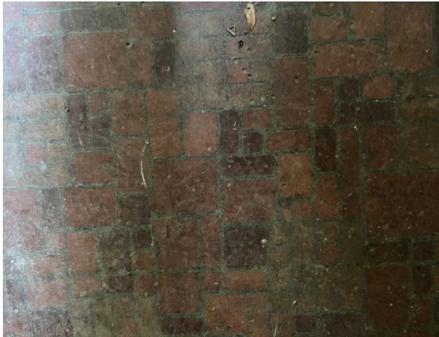
Figure 48. Decorative vinyl flooring in kitchen.
