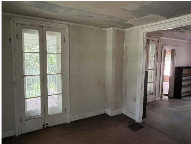
Figure 38. Chase in southeast corner of parlor.
