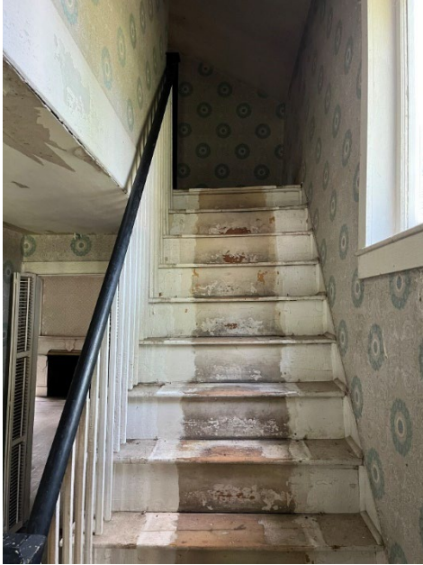
Figure 35. Wood stair in front hall.
