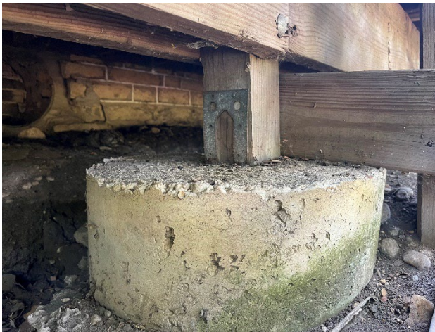
Figure 11. Wood framing and concrete piers at wrap-around porch.
