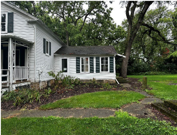
Figure 4. Concrete-paved walks adjacent to house. (Source: All photographs by WJE, 2024, unless otherwise noted)
