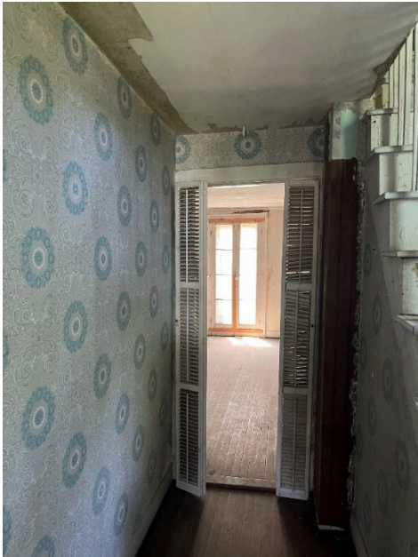
Figure 37. Chase on south wall of front hall.
