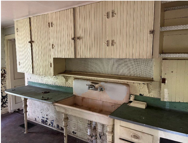
Figure 54. Built-in countertops, wood cabinets, and painted cast iron sink.
