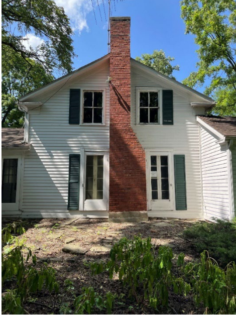
Figure 21. South facade of the main house.
