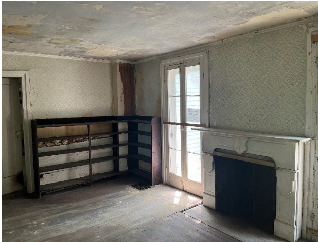
Figure 39. Fireplace and chase on south wall of living room.
