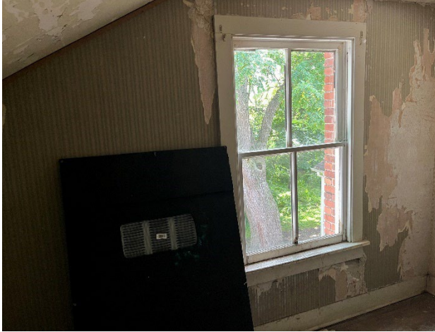
Figure 62. 2-over-2 Double-hung windows at second floor.
