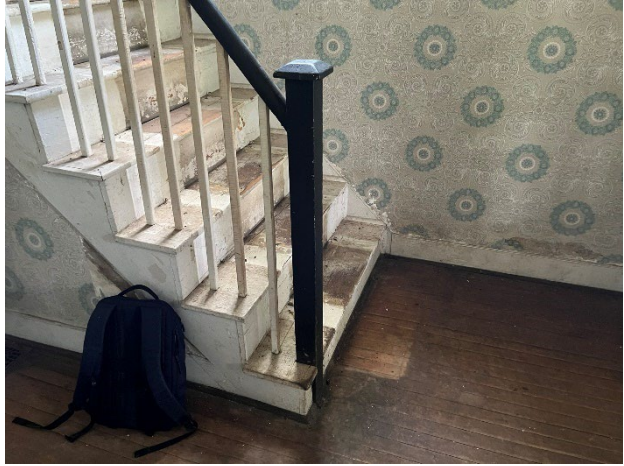
Figure 36. Decorative balustrade at wood stair in front hall.
