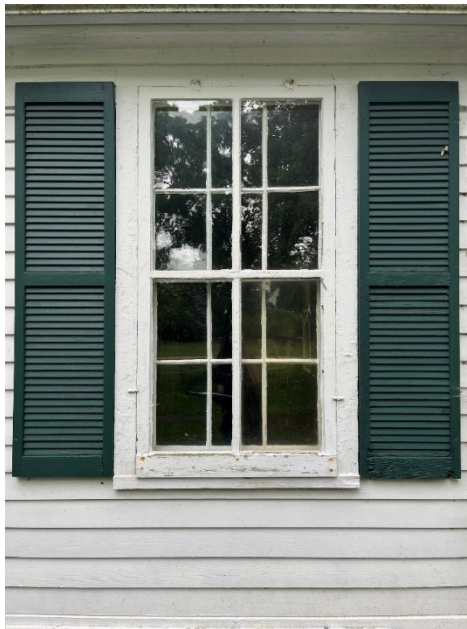
Figure 16. Typical six-over-six wood window with two-over-two storm window.
