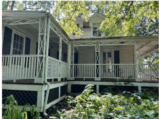
Figure 20. Partial view of east facade of the main house.
