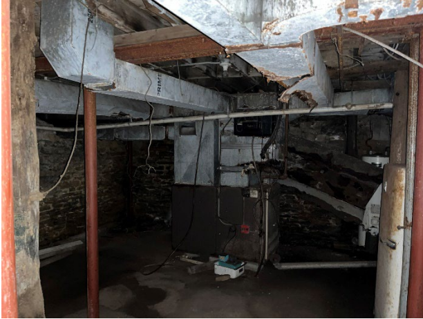
Figure 70. Basement from northwest corner.
